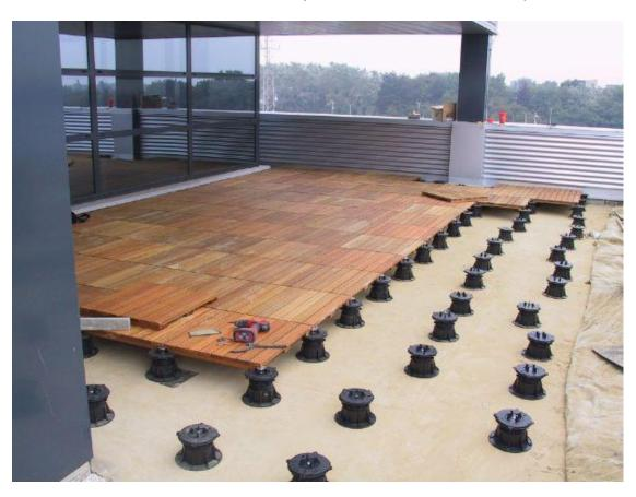
3) Once the tiles are laid out and leveled you can attach our wood fastening
