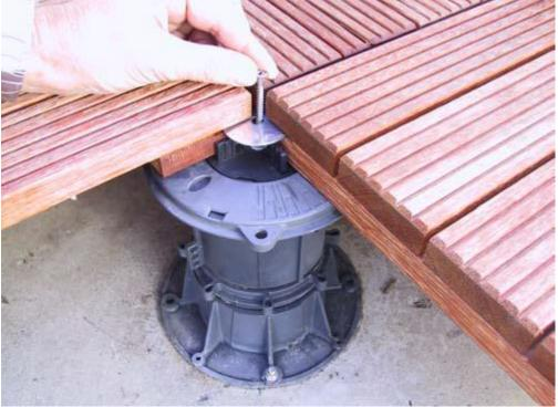
5) Tighten the screw just enough to lock the tiles in place, (you will go back to each screw and do a final tightening once all the tiles are in place. You will need a
