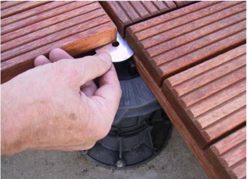
4) Slip a 1 inch stainless screw down into the middle of the washer and spacer tab underneath.
